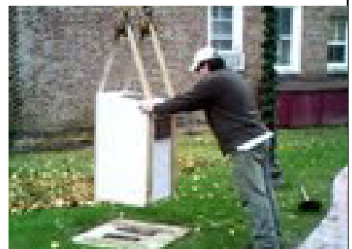
Monument being put into place at CT
